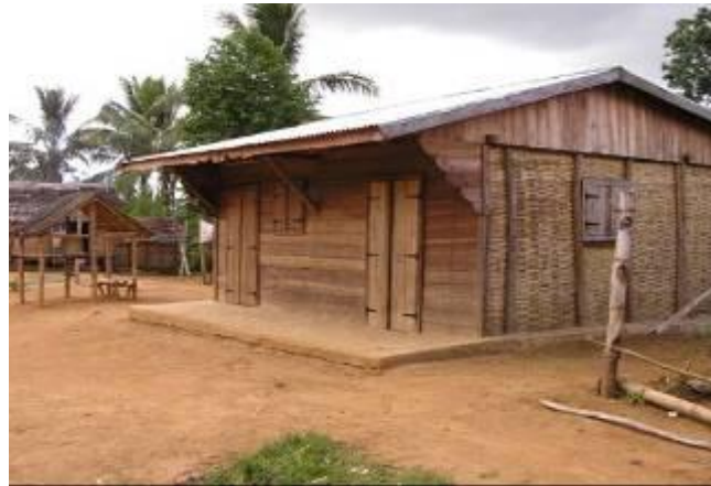
Figure 25: Semi-hard construction in Vavatenina
