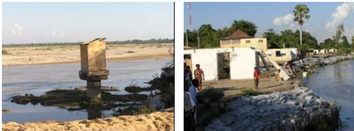
Figure 34: Market building in Mahabo
