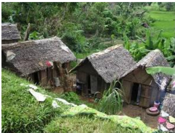
Figure 26: Local materials construction in Sainte-Marie
