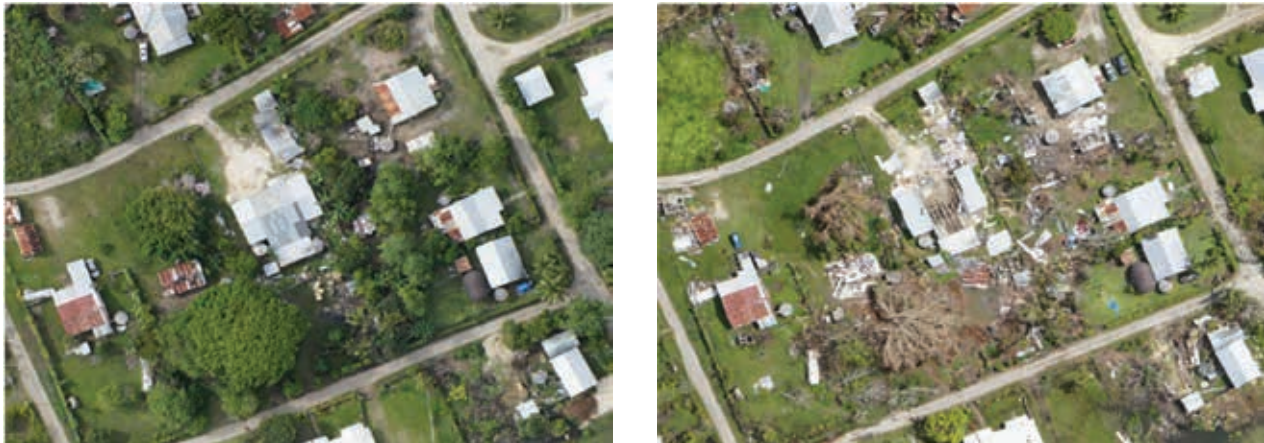
FIGURE 15. Images showing pre- and post-event status of the same structures.
