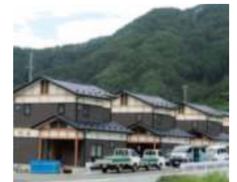
Public housing under construction (Otsuchi Town, September 2014)
