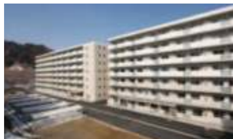
Public housing for survivors in Heita, Kamaishi City (completed on January 24, 2015)
