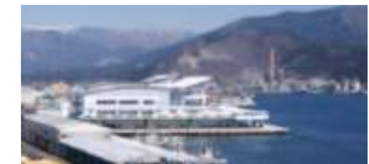
Development of a fish market with advanced hygiene management (Ofunato Fish Market, completed in April 2014)
