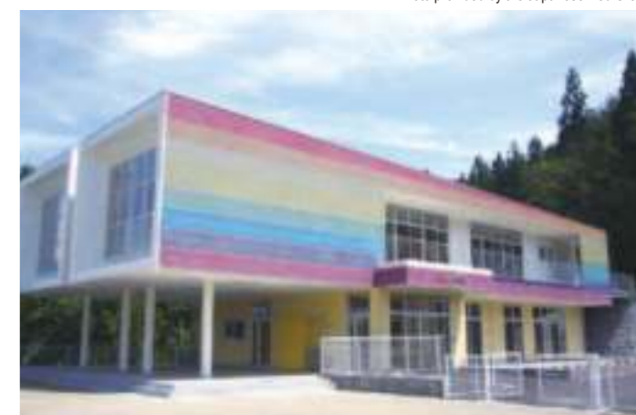
Daycare center built with international donations (Otsuchi Town, August 2014)
