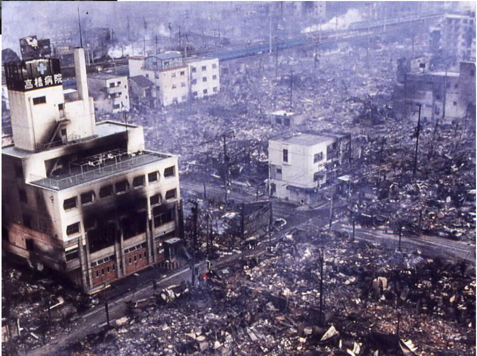
Fire in residential area (Suma Ward)
