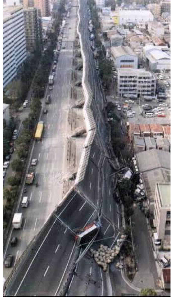
Collapse of Hanshin Expressway (Higashinada Ward)
