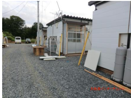
Additional work to attach heat insulation panel.
