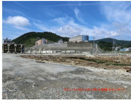
Hospital on the hill 15m high from sea level. Tsunami attacked the first floor.
