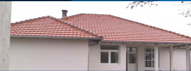
Elementary school Kalinovac - UB
